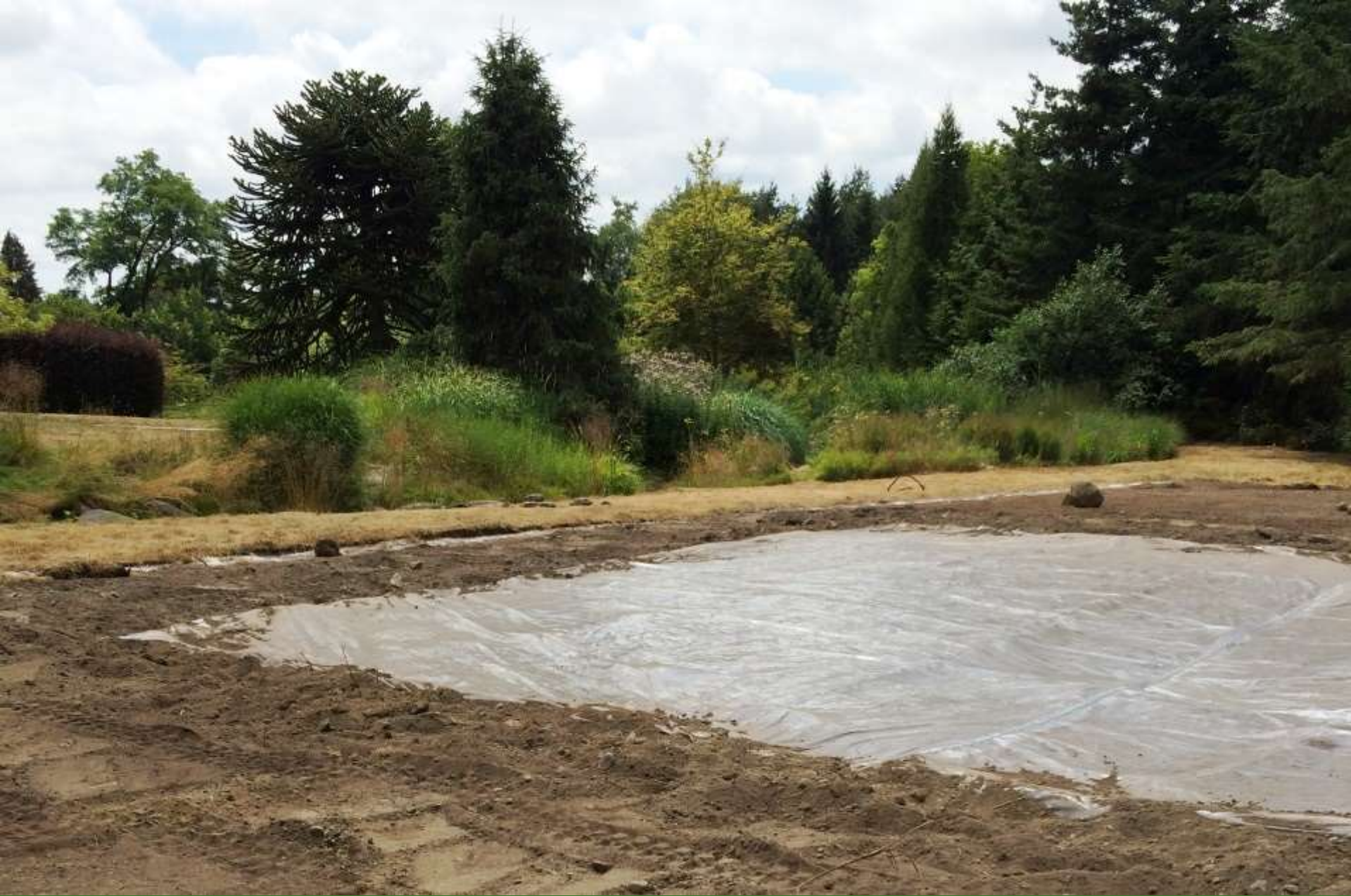
Filled in trench
